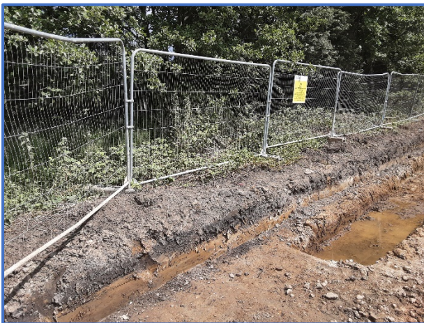
Photograph 3: Excavation within RPAs of Group G4.
