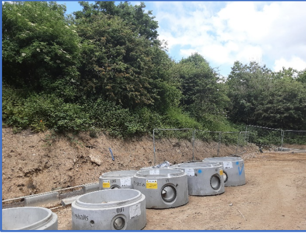
Photograph 8: Additional Shrubs and young Trees retained.
