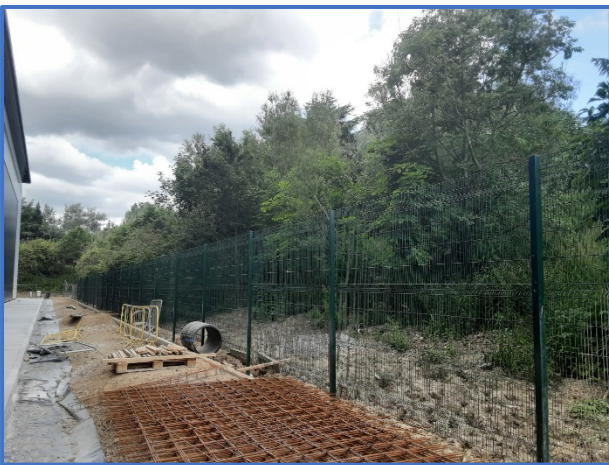
Photograph 7: New Site Boundary Fence.
