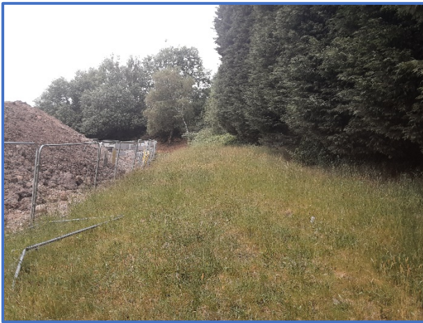
Photograph 2: Tree Protection Fencing around Group G2.
