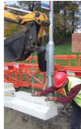
Installation made safe & Easi
