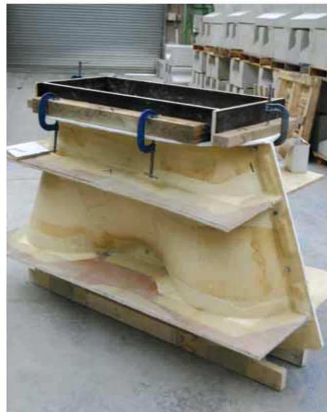
Pre-cast concrete angled column bases of new apartment block in Stalybridge
