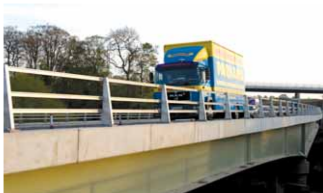
New River Wharf Bridge A1(M) Wetherby
