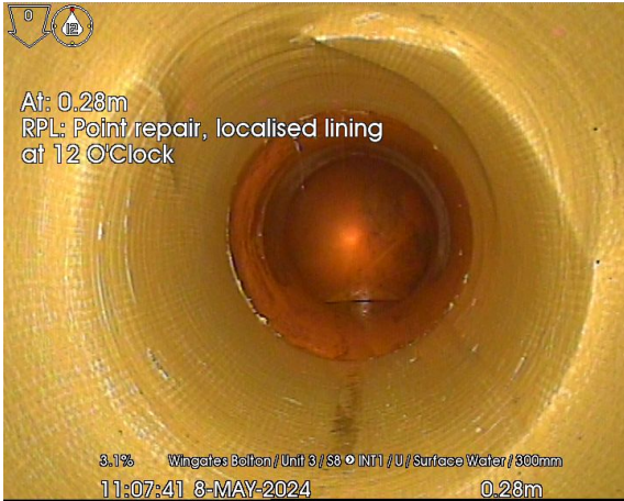
S8 - INT1_0-28m_110741.jpg, 00:00:08, 0.28 m Point repair, localised lining at 12 o'clock
